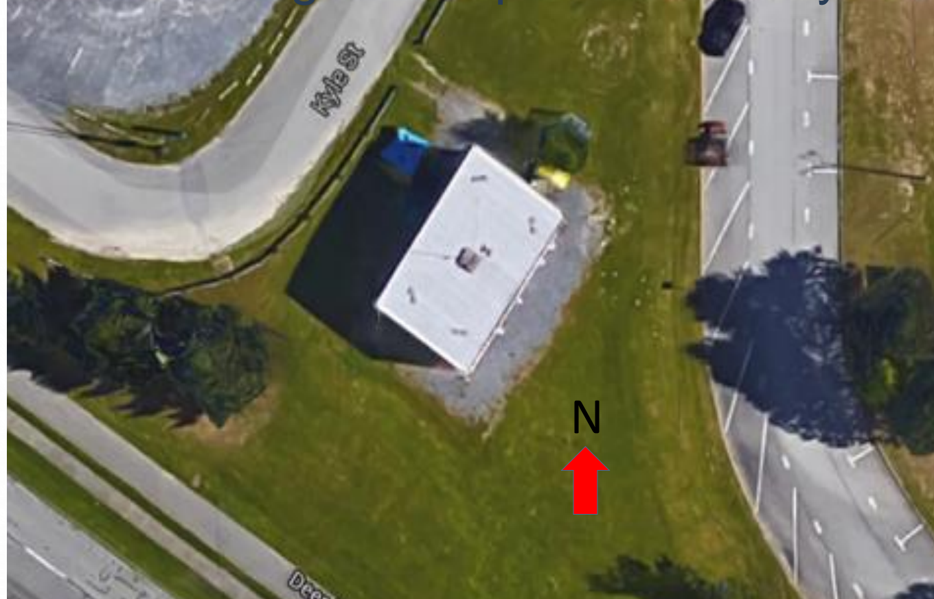
Building Envelope Test Facility at BCIT Campus. (Google Maps, 2015)
