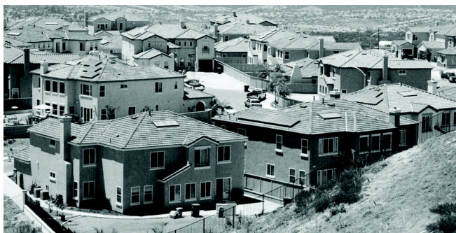
Figure 2 Neighborhood installations of solar thermal and electric collectors.
