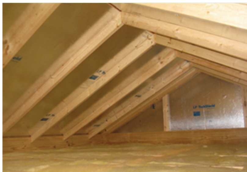
Figure 3 Test attic with low-e foil laminated on OSB.
