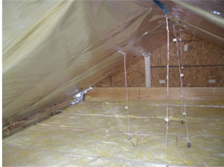
Figure 4 Test attic with low-e foil stapled on rafters.
