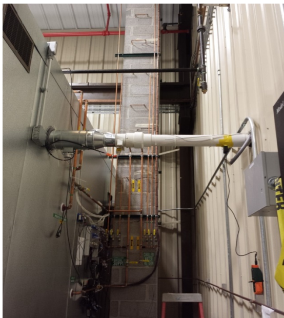
Fig. 14. Round duct for control of pressure in the room and measurement of combustion/dilution makeup air.
