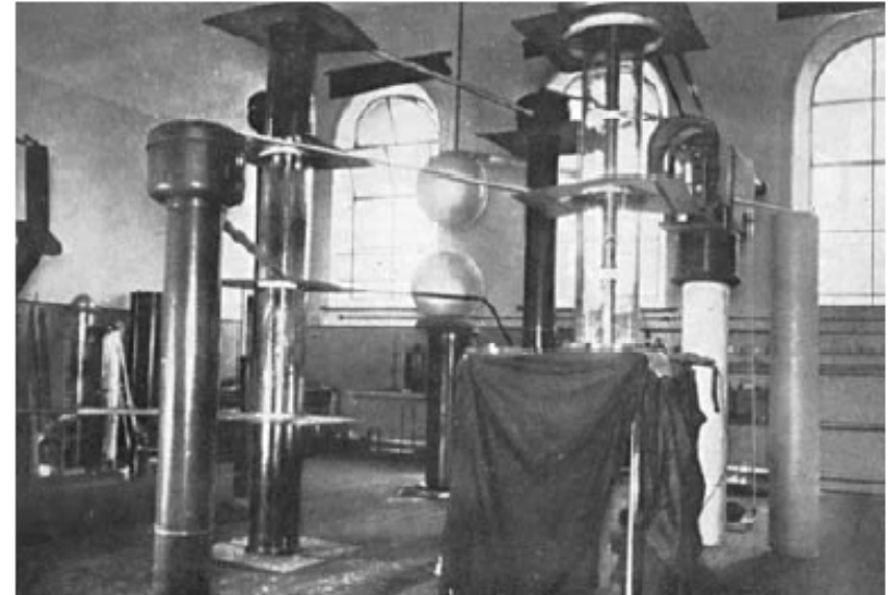
Cockroft and Waltons 800 kV accelerator, Cavendish Laboratory, Cambridge, 1932
