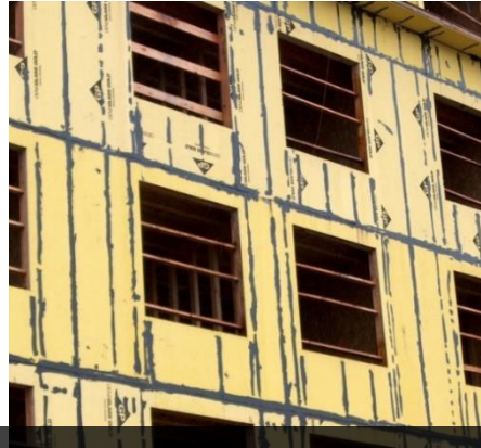
Sealed Gypsum Sheathing – Sealant Filler at Joints
