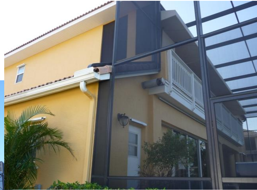
NW corner view
