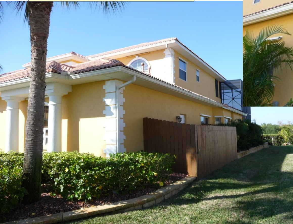
NE corner view
