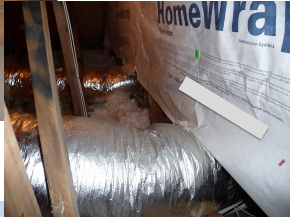
West side attic view
