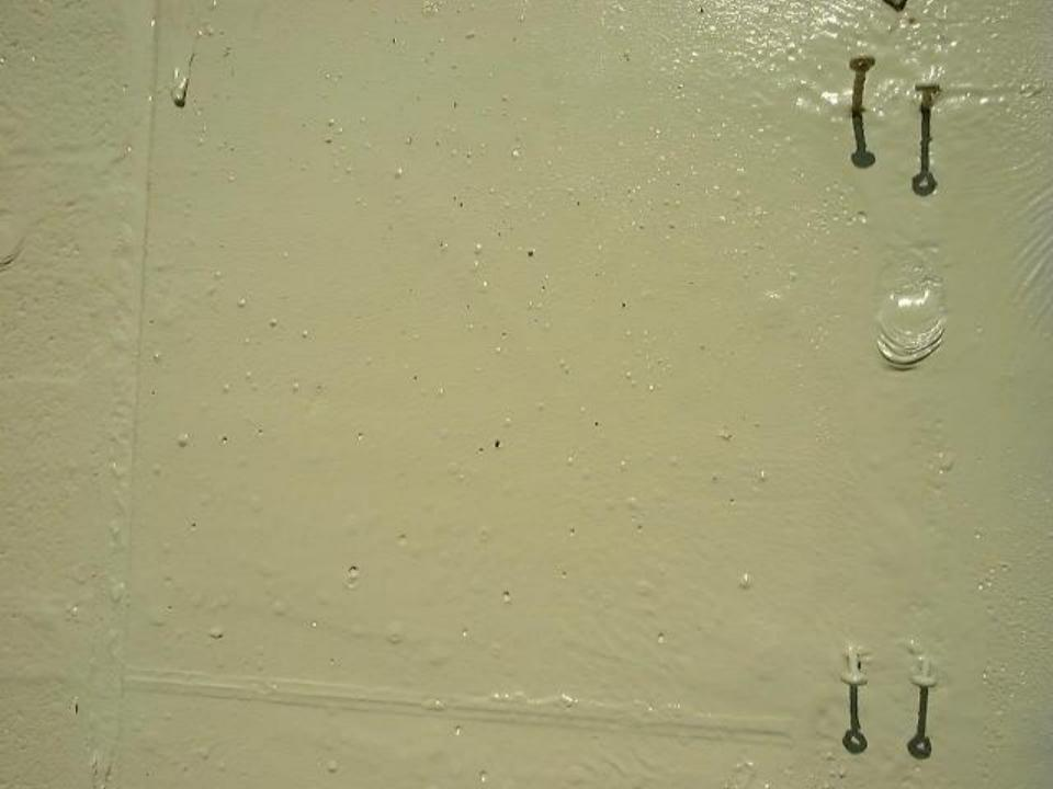
Craters from air in the equipment or contaminated materials from improper cleaning of the equipment results in air leakage
