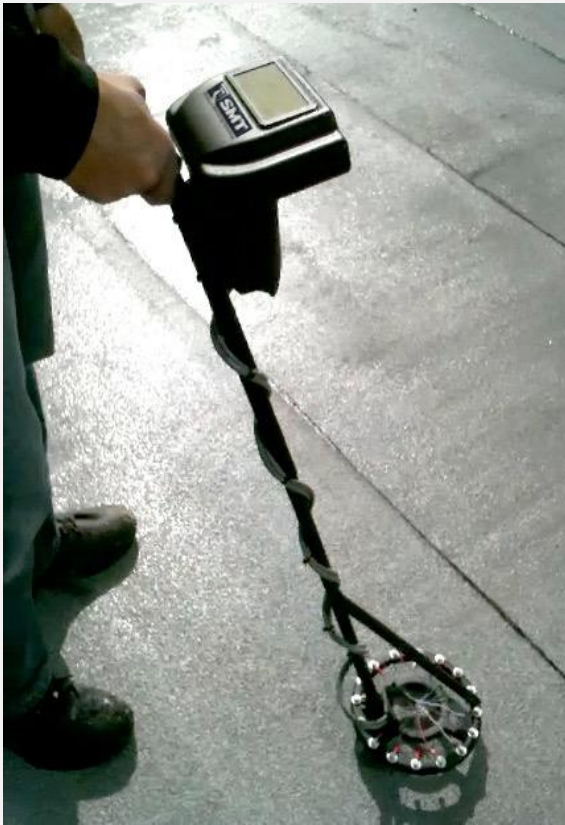
Immediately after membrane installed.
