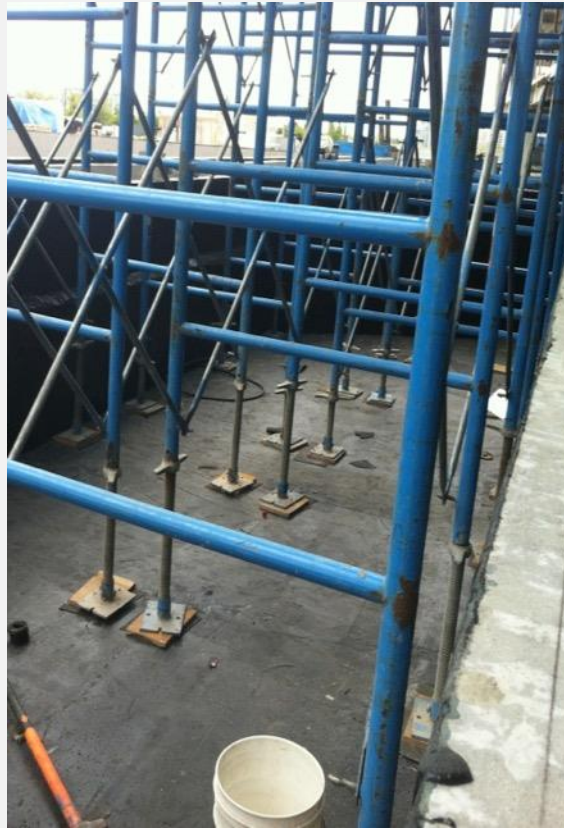
Prior to covering with overburden.
