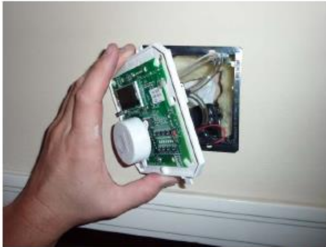
Figure 7-23: Typical SMT-A3 unit being installed in a wall above a suite entrance door
