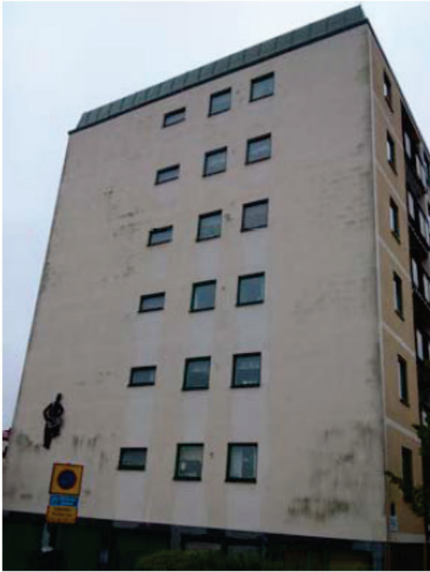
Figure 8 Left: appearance of MBG on retrofitted façade. Right: MBG removed from the façade by water.
