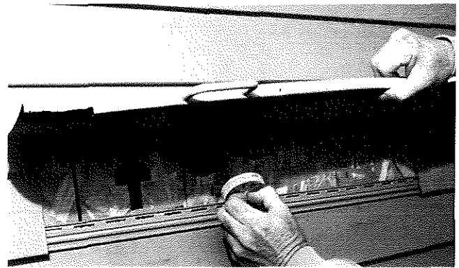
Figure 3 Test building wall with removable plug.
