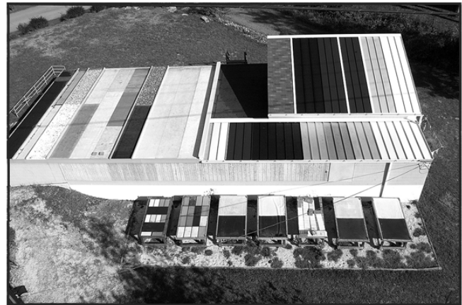
Figure 1 The Envelope Systems Research Apparatus used for testing painted and unpainted metal roofing.
