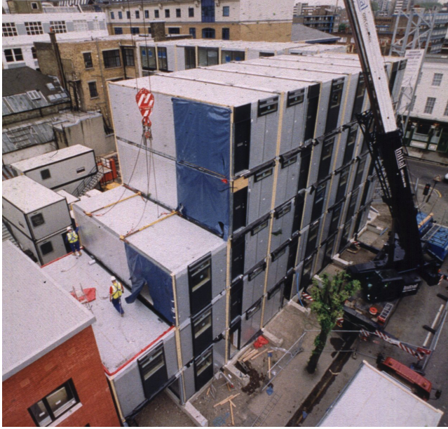
Figure 2 A volumetric housing scheme under construction in London.
