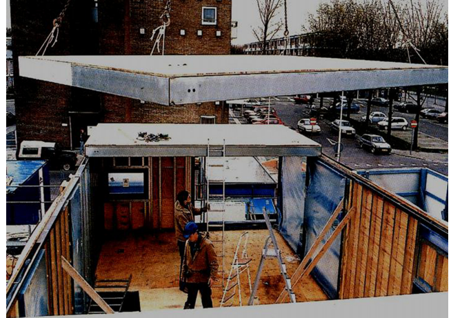
Figure 3 Light steel frame panellized construction.
