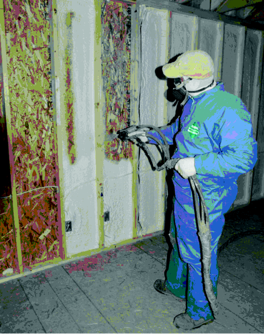
Figure 7 Application of closed-cell foam insulation.
