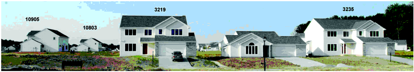
Figure 1 View of houses from the north.
