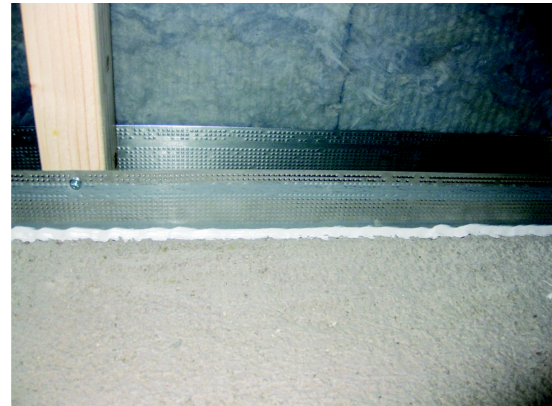
Figure 15 An example of an airtight connection to the floor. The polyethylene film runs behind the services gap, underneath the steel joist (to which flexible bottom plate insulation is adhesively bonded), and is then bonded to the concrete.
