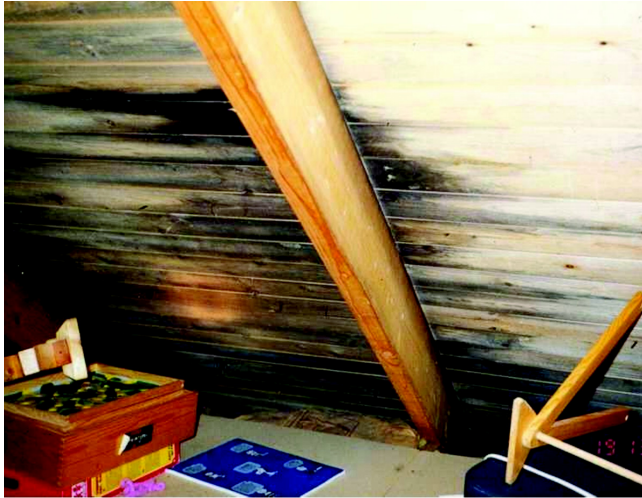
Figure 1 Mold growth in a cold attic.
