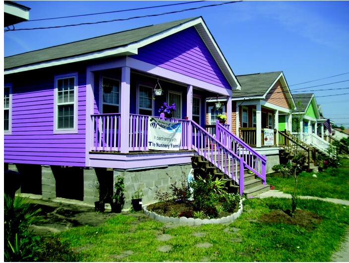
Figure 1 Houses with pier foundations recently constructed by Habitat for Humanity in New Orleans, Louisiana.
