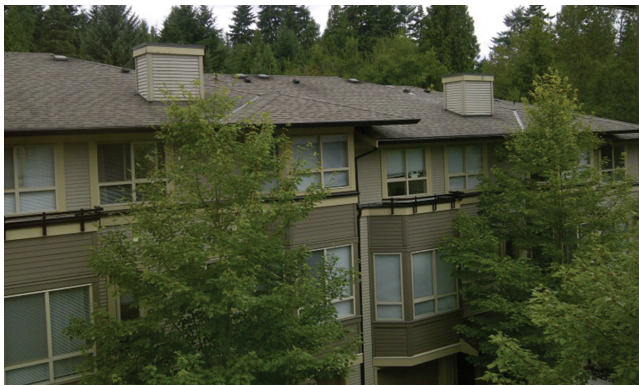
Figure 5 East elevation of Unit 1.
