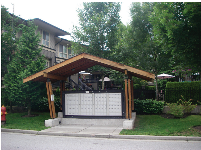
Figure 6 Test (control) roof assembly with Unit 2 in the background.
