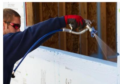
**Figure 1. The sprayable liquid flashing can be applied with a regular professional paint sprayer, roller or brush.**
