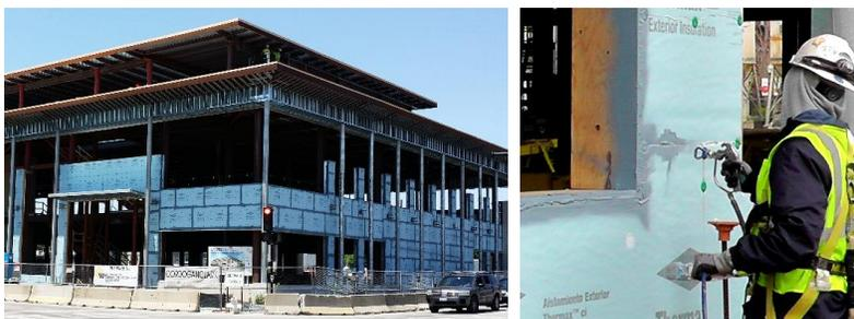
Figure 4. Demonstration building with liquid flashing sealing the gaps around penetrations and joints between THERMAX boards.
