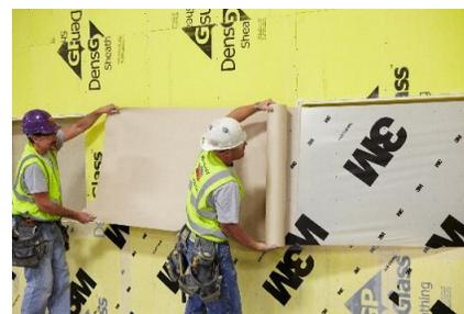
**Figure 2. The primer-less self-adhered membrane can be installed on most construction materials without a primer.**
