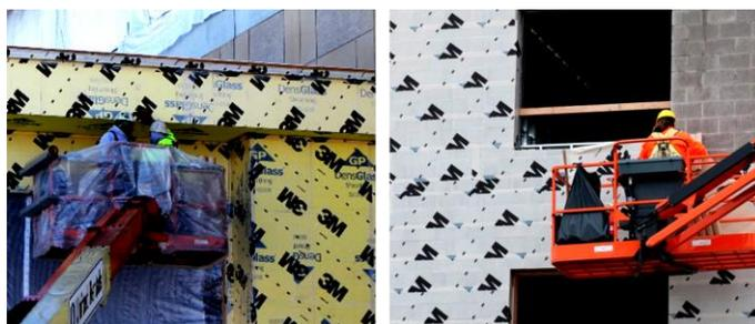
Figure 5. Demonstration buildings with the primer-less self-adhered membrane on DensGlass and concrete masonry blocks.
